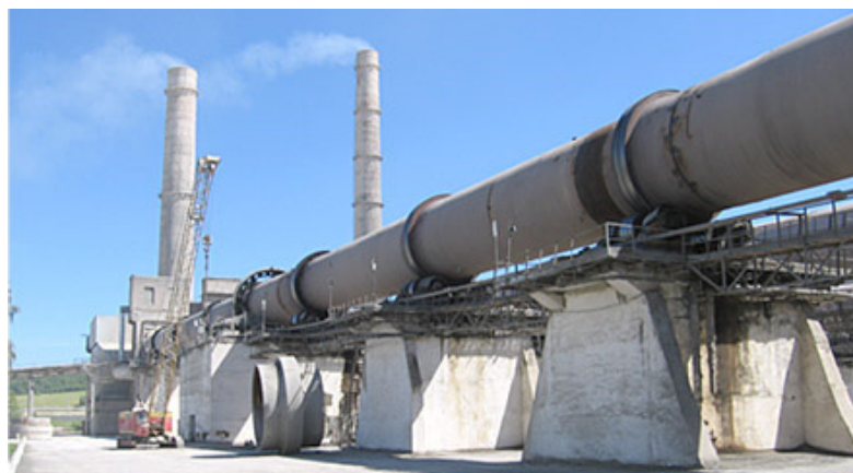
Fig. 1. Outward appearance of a cement kiln [6].
