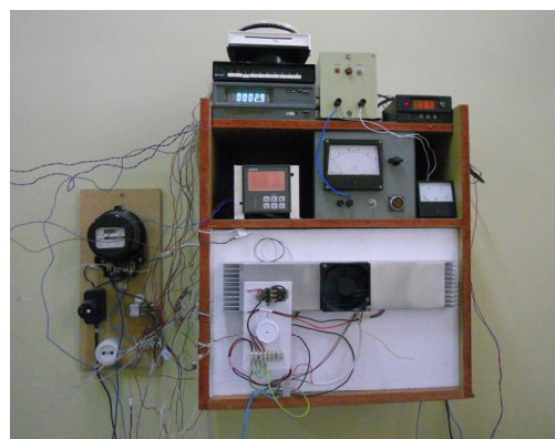
Fig. 1. Transport thermoelectric cooler (as seen from thermoelectric unit) during the test.
